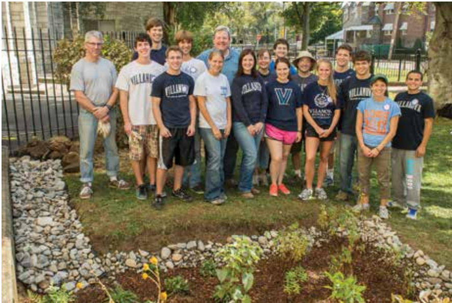
On Villanova's annual St. Thomas Day of Service, faculty and students helped to design and install a rain garden at St. Martin of Tours School in Philadelphia.
